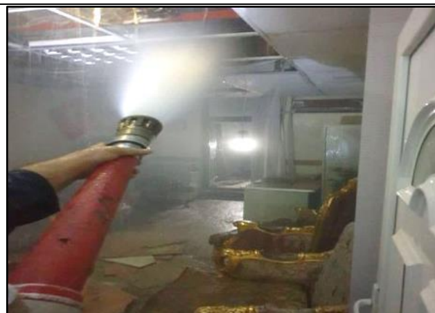
Figure 14. Extinguishing the secondary ceilings that led to the spread of the fire.
